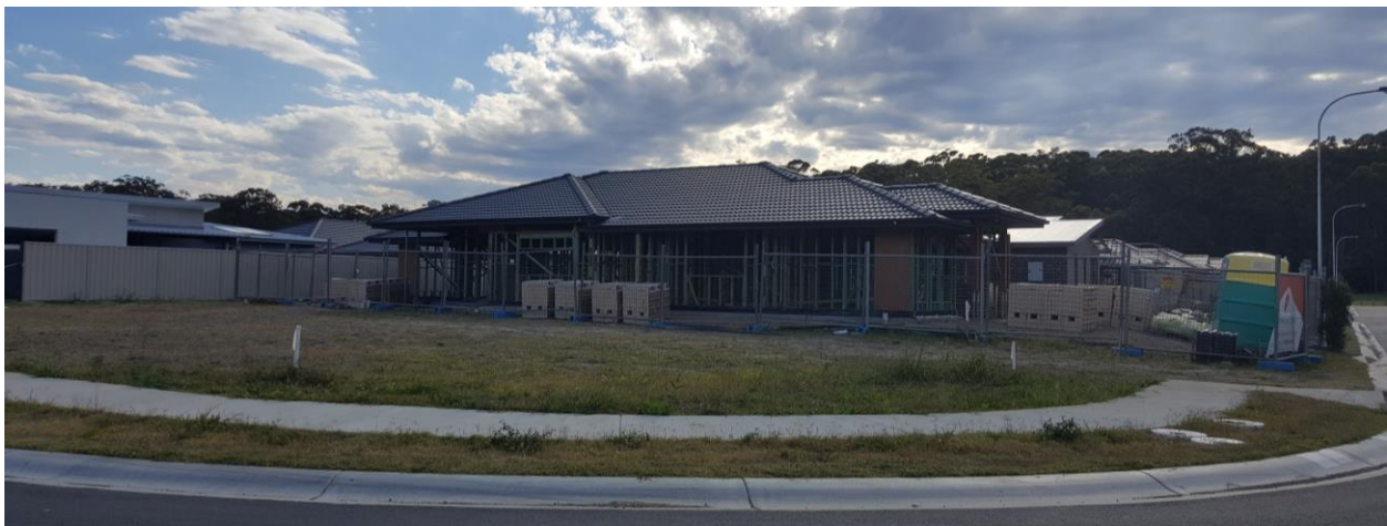
Detached housing construction at North Sandy Beach
